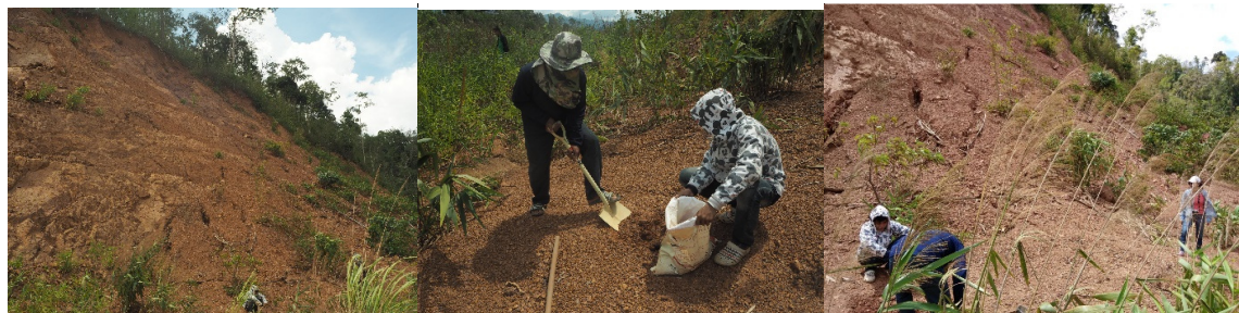
Location of Laterite at Sta.102+400
