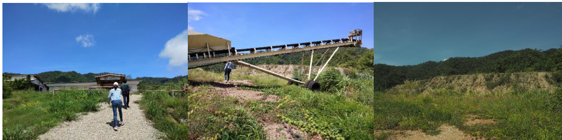
Location of Rock at Sta.145+300
