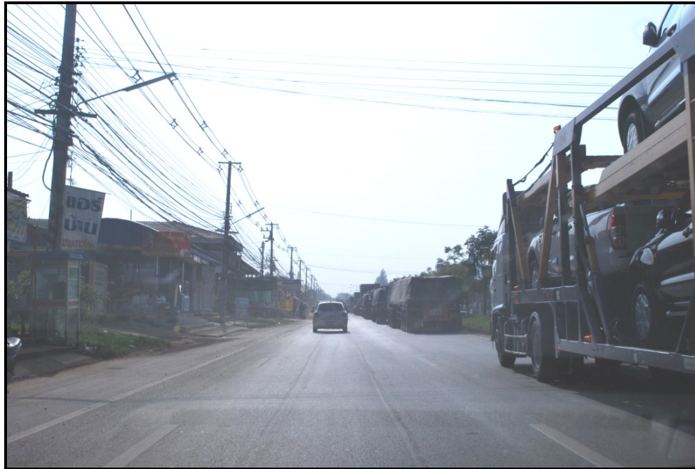
Figure 4.4 Physical Characteristic of National Highway No. 33 of Thailand (eastbound)
