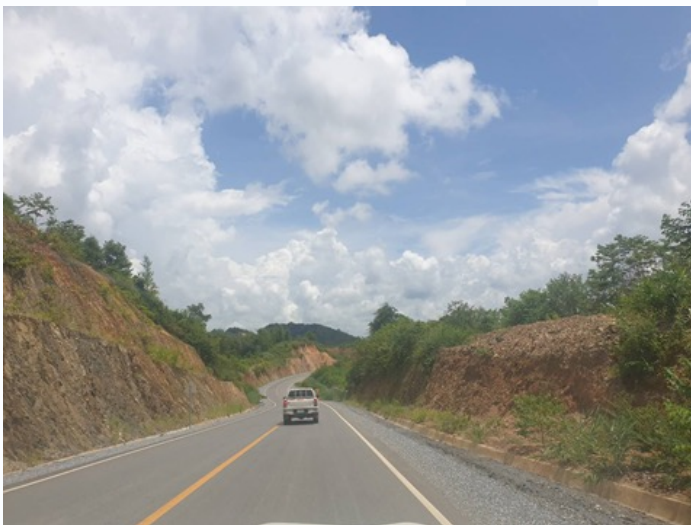
Route conditions under construction under the R11 project
