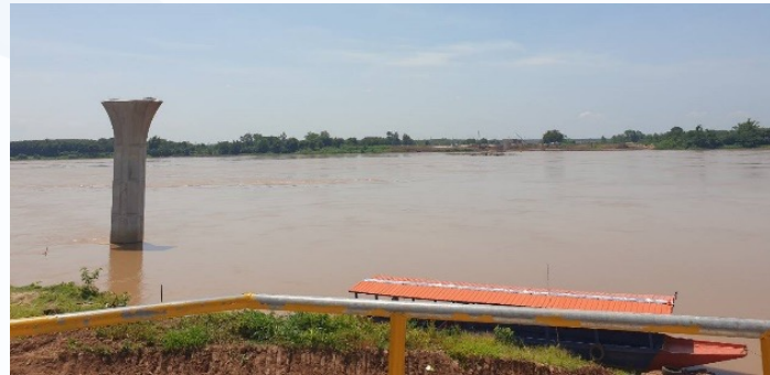
Construction site of the 5th Friendship Bridge
