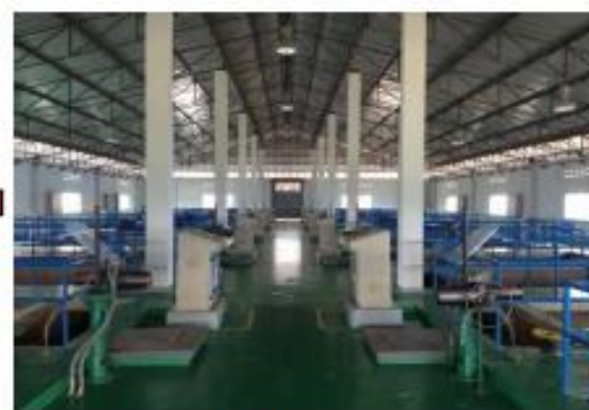
Filtration (Rapid sand filtration)
