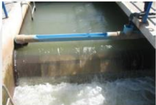
Coagulation (Rapid mixing) (mixer cone)
