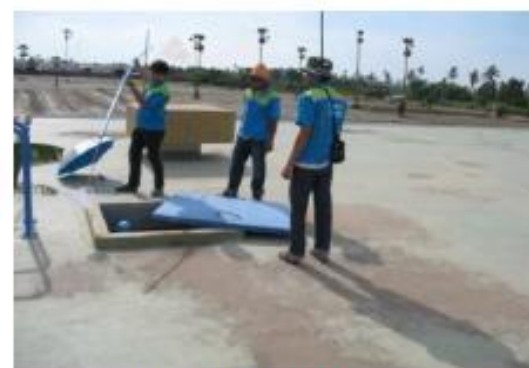
Clear water tank
