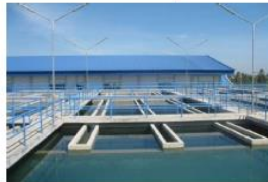
Sedimentation (Rectangular sedimentation tank)
