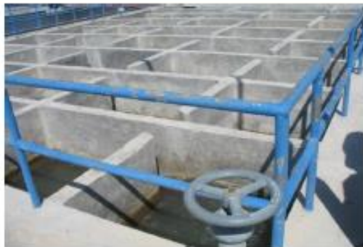
Floculation (Slow mixing) (Horizontal baffled flocculator)
